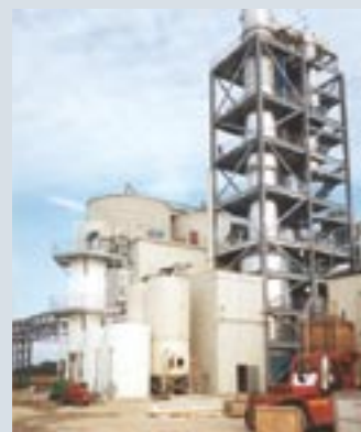
This soybean processing plant recently installed the fieldbus system as part of a plant expansion.
